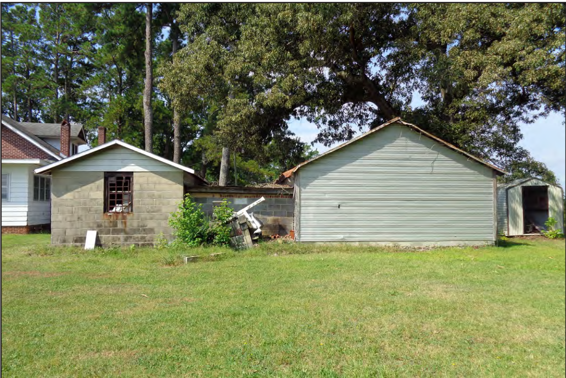
PLATE 14: 655 Longbranch Road Garage and Connected Shed, Looking Southwest
