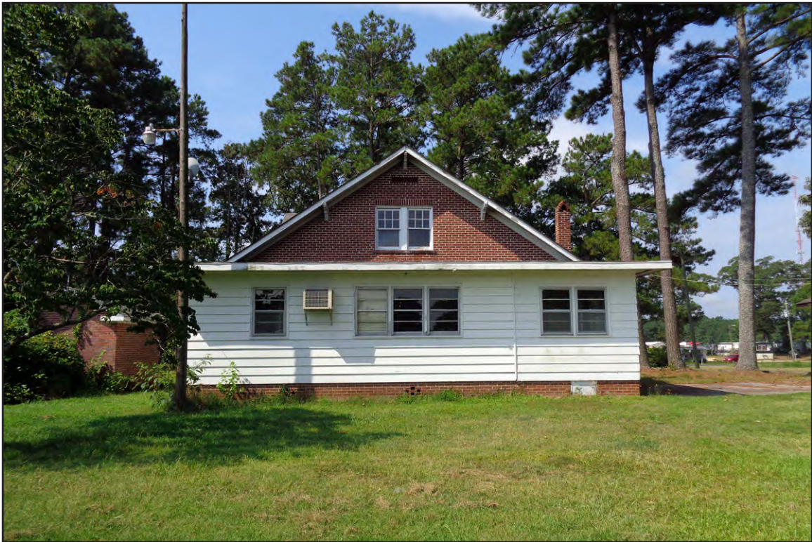
PLATE 10: 655 Longbranch Road Dwelling Northeast Elevation, Looking Southwest
