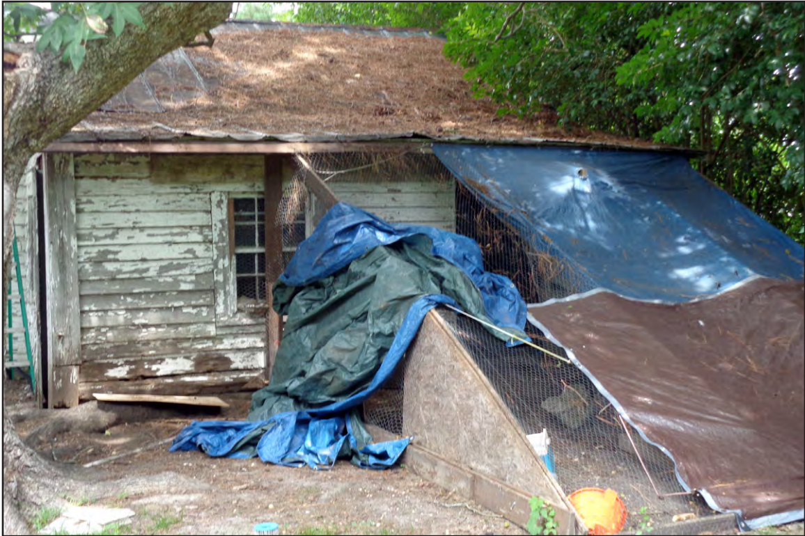
PLATE 34: 3359 Bud Hawkins Road Dwelling Wood Shed South Elevation, Looking Northeast
