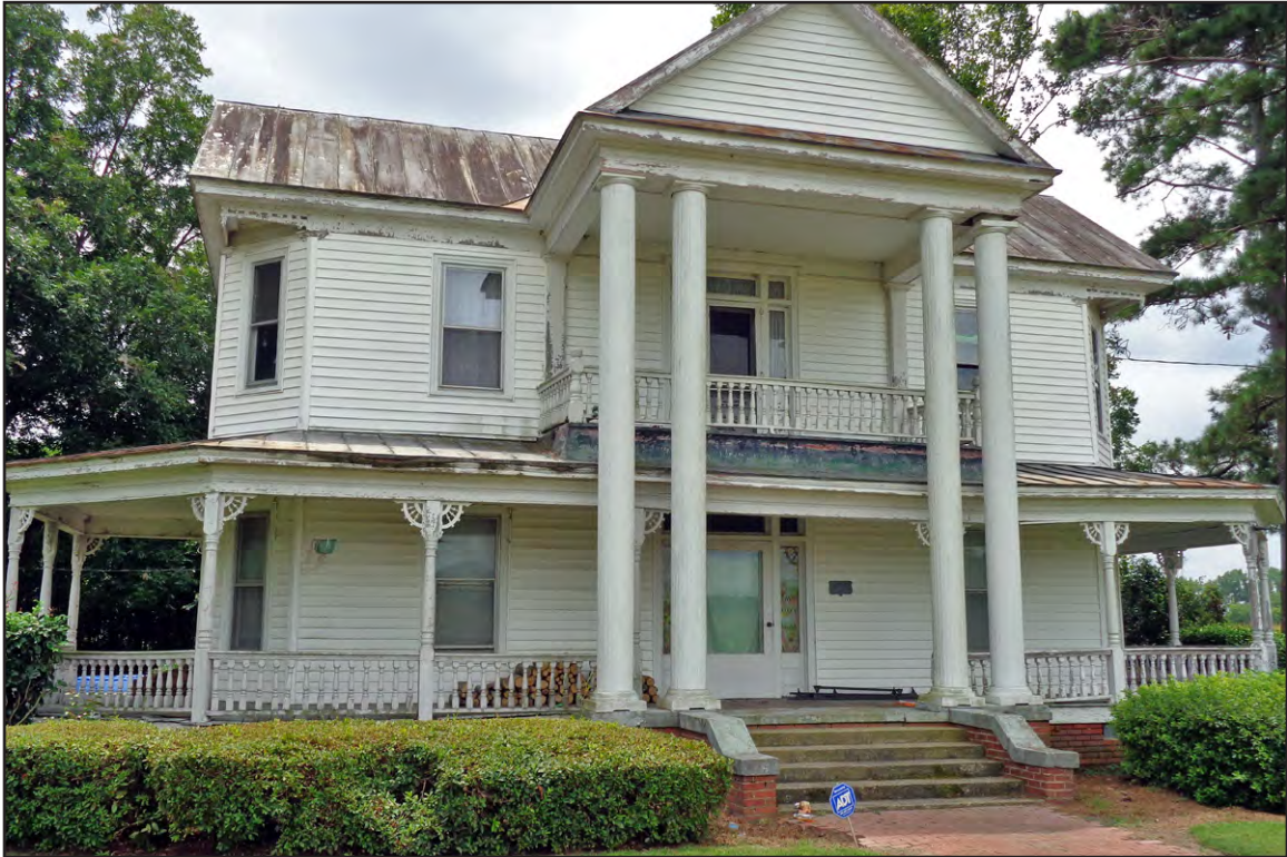
PLATE 22: 3359 Bud Hawkins Road Dwelling North Elevation, Looking South
