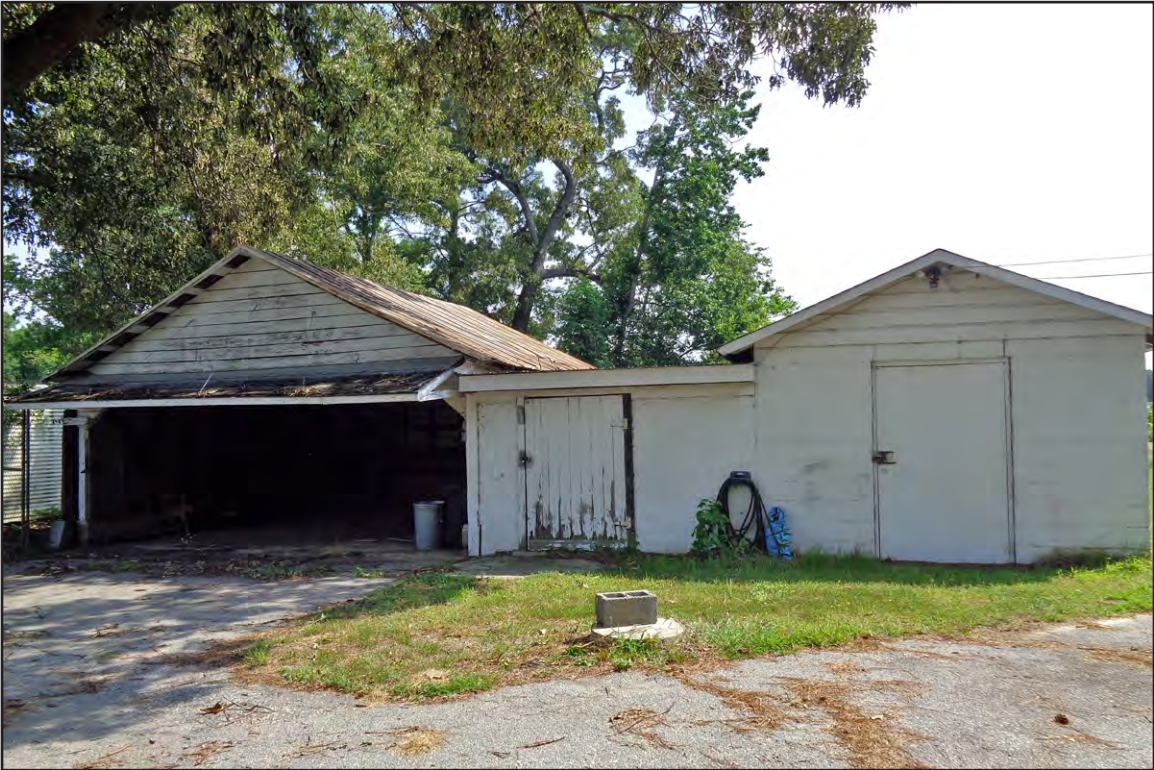
PLATE 13: 655 Longbranch Road Garage and Connected Shed, Looking North
