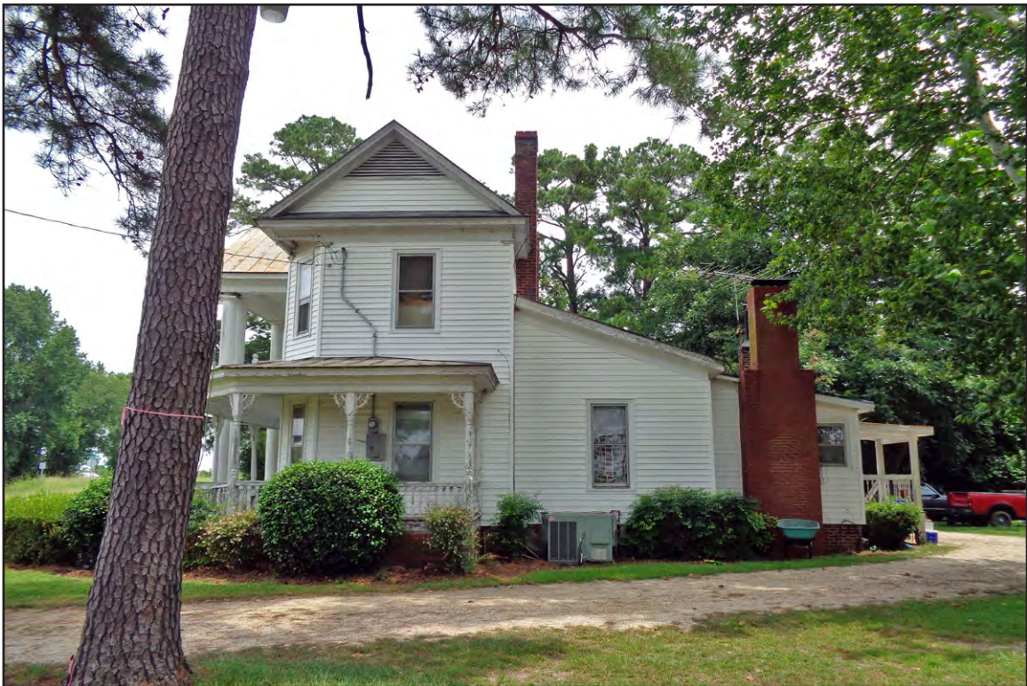
PLATE 23: 3359 Bud Hawkins Road Dwelling West Elevation, Looking East
