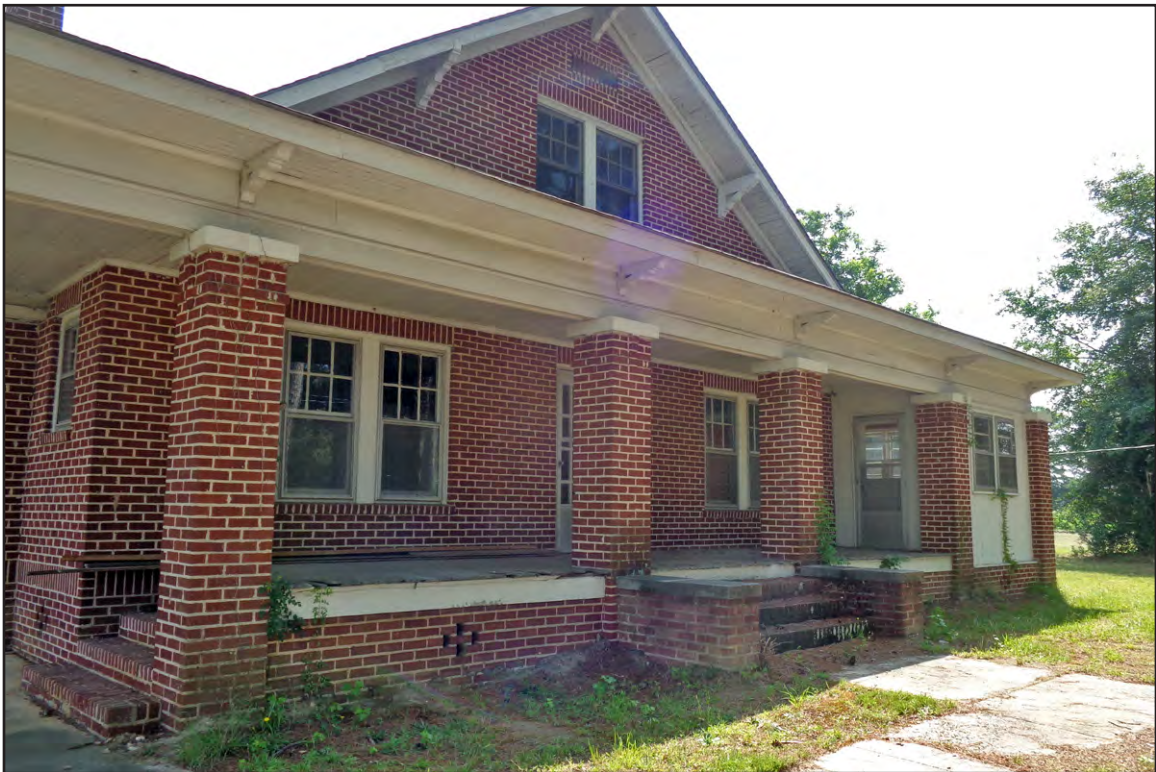
PLATE 4: 655 Longbranch Road Dwelling Porch, Looking East
