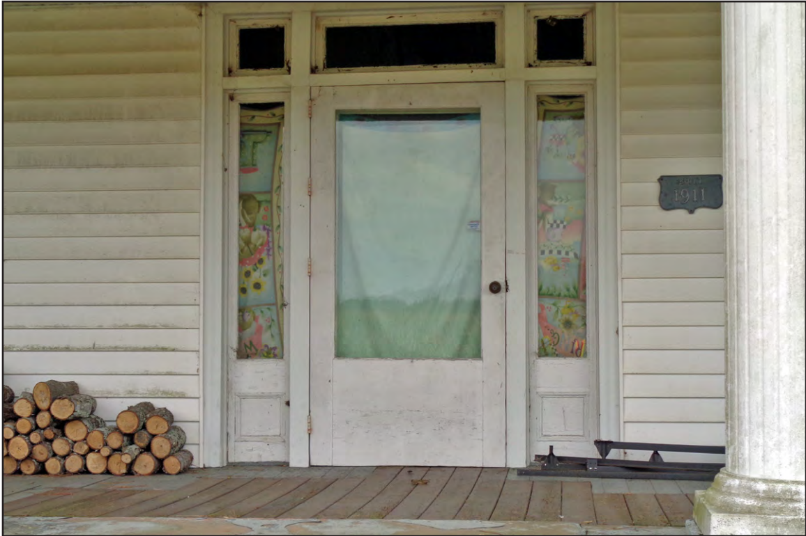
PLATE 28: 3359 Bud Hawkins Road Dwelling Entrance Door, Looking South
