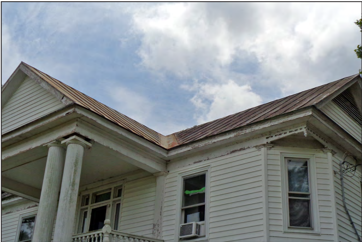
PLATE 29: 3359 Bud Hawkins Road Dwelling Façade Windows
