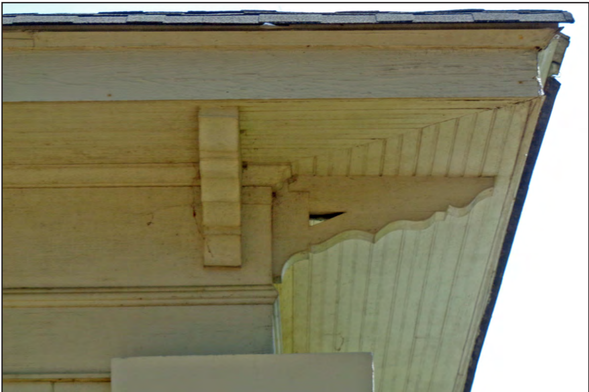
PLATE 6: 655 Longbranch Road Dwelling Bracket and Soffit Detail
