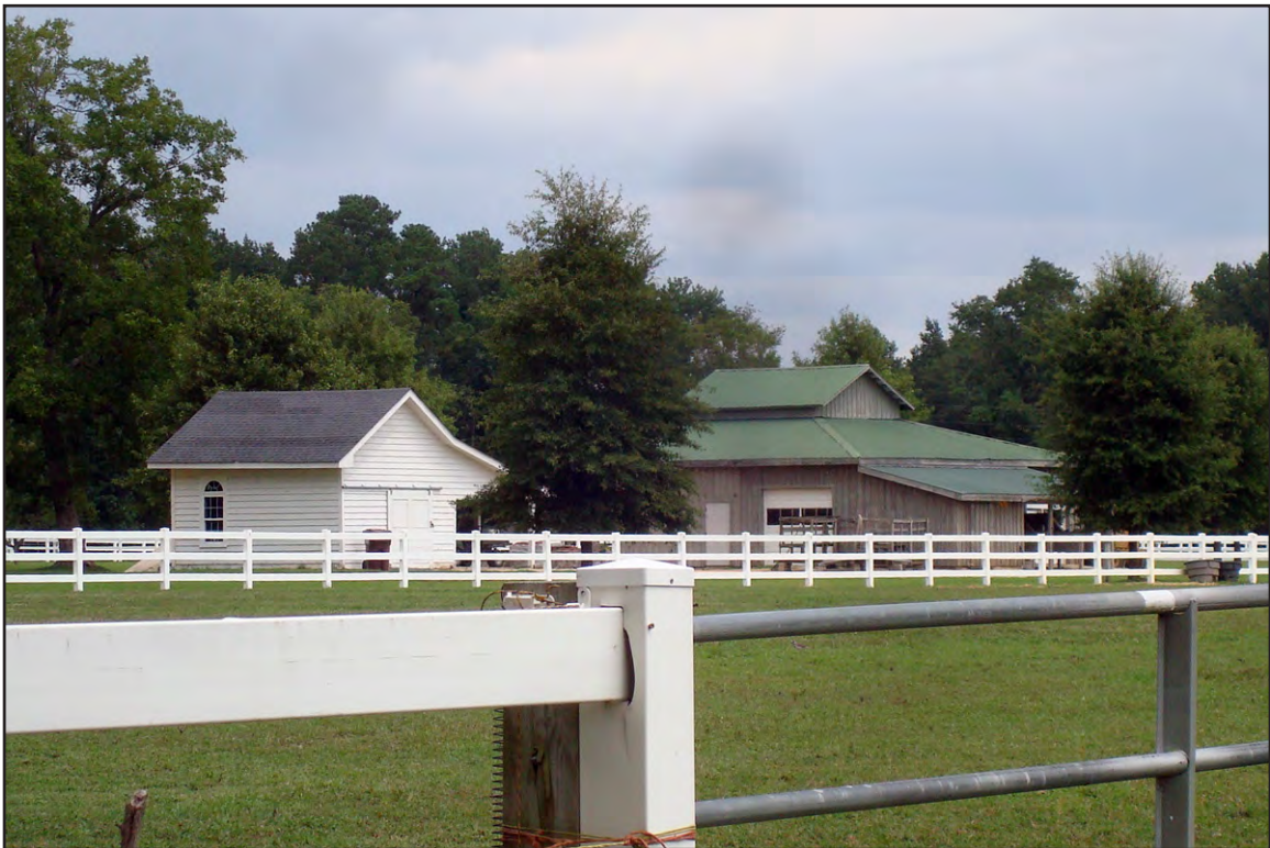
PLATE 18: Ivy Burne (HT0024) Farm Complex, Agricultural Outbuildings, Looking Northeast
