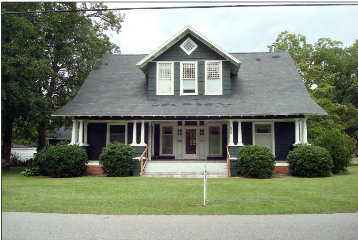
PLATE 19: Thompson-Pope House (HT0418), Façade, Looking Northwest
