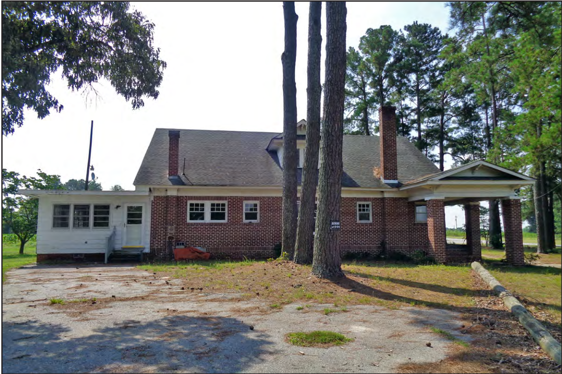
PLATE 5: 655 Longbranch Road Dwelling Northwest Elevation, Looking Southeast
