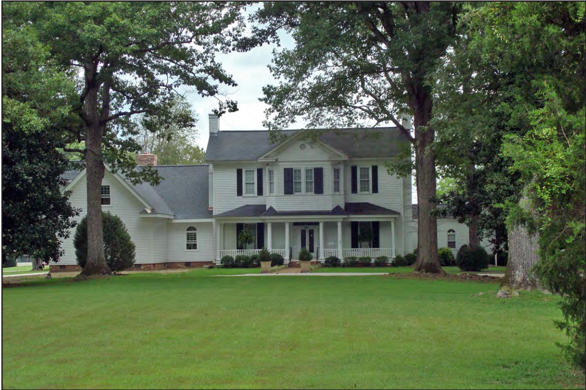
PLATE 17: Ivy Burne (HT0024) Farm Complex, Façade, Looking East
