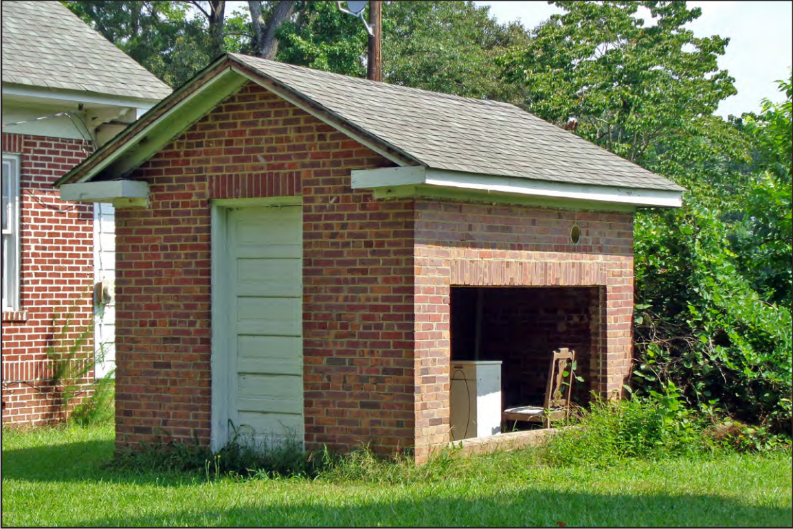
PLATE 15: 655 Longbranch Road Brick Outbuilding, Looking North
